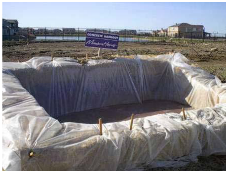
Plate 2.1: Example of a Temporary Concrete Washout Area
